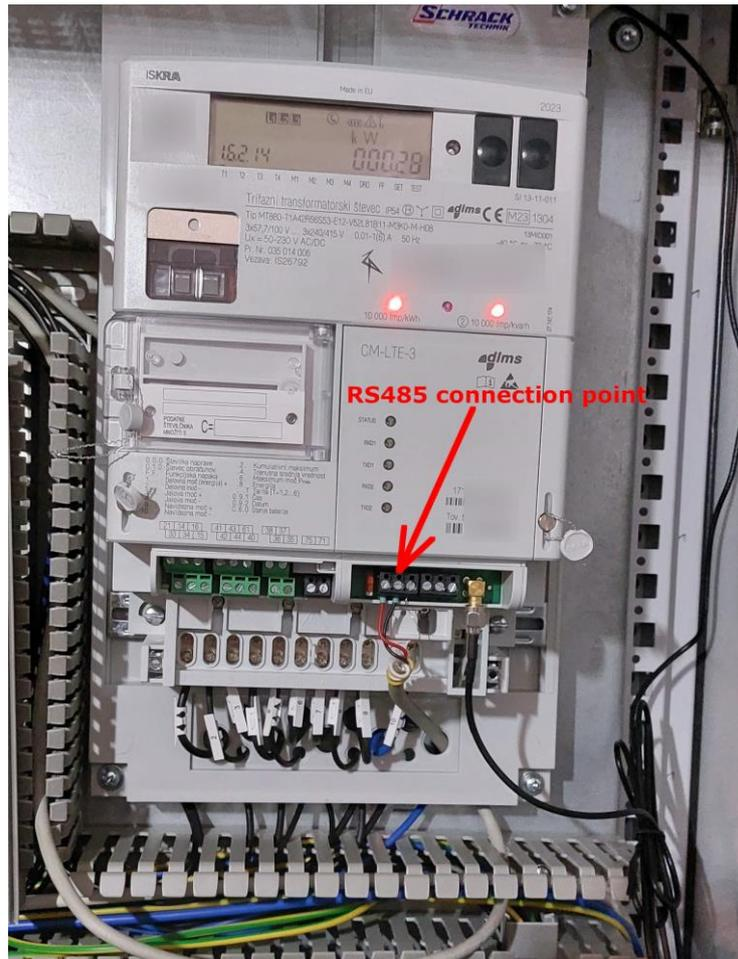
Figure 14: Connection to the industrial DSO electricity meter Iskraemeco via RS485 one-way (half-duplex) and DLMS/COSEM communication protocol
