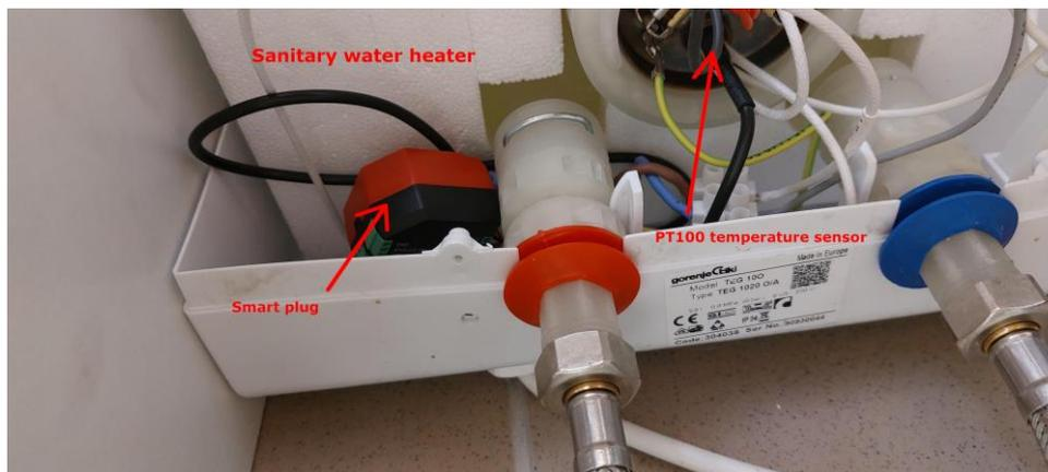
Figure 12: Installation of a smart socket and temperature sensor PT100
