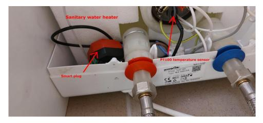
Figure 12: Installation of a smart socket and temperature sensor PT100
