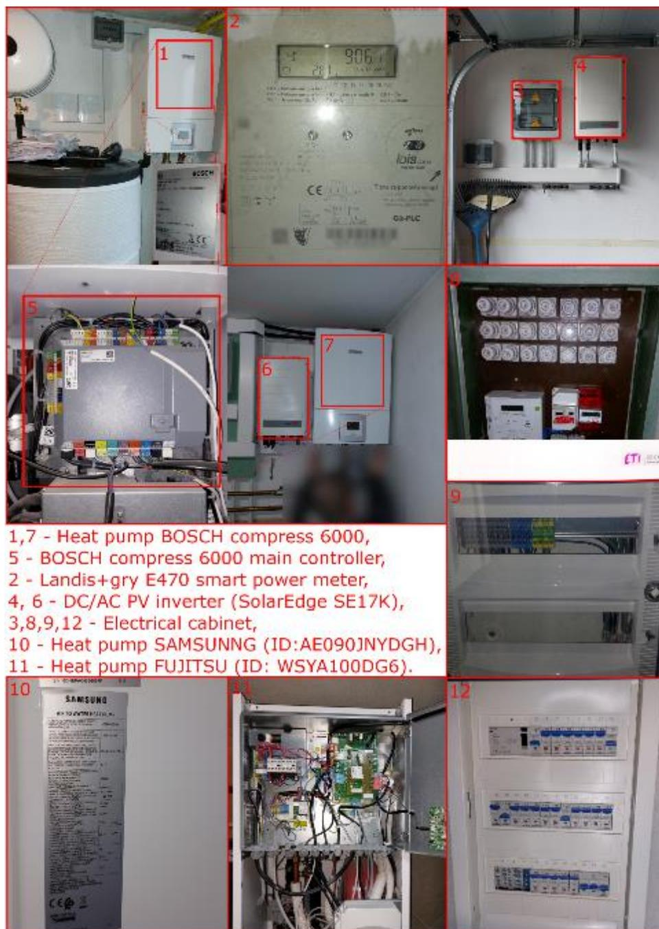
Figure 6: Build-in equipment in houses of first pre-pilot users
