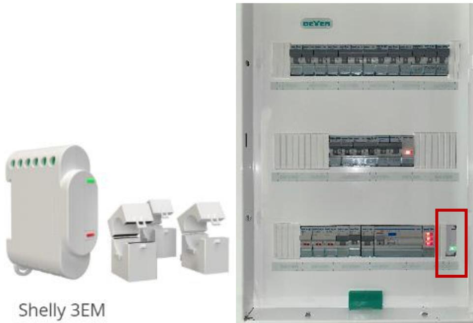
Figure 1: The Shelly Smart Meter and the installation in the user's electrical board
