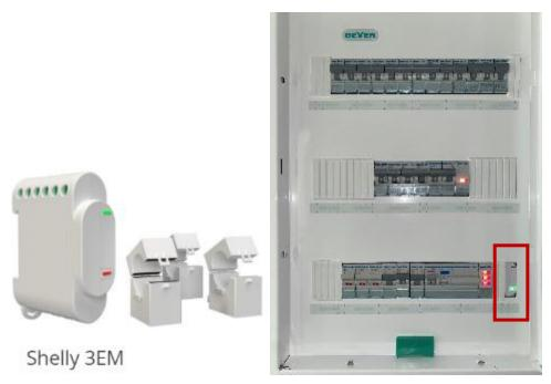
Figure 1: The Shelly Smart Meter and the installation in the user's electrical board
