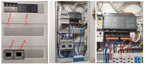
1. Protective fuses (3x20 A for solar power plant and 1x5 A for HEMS),
