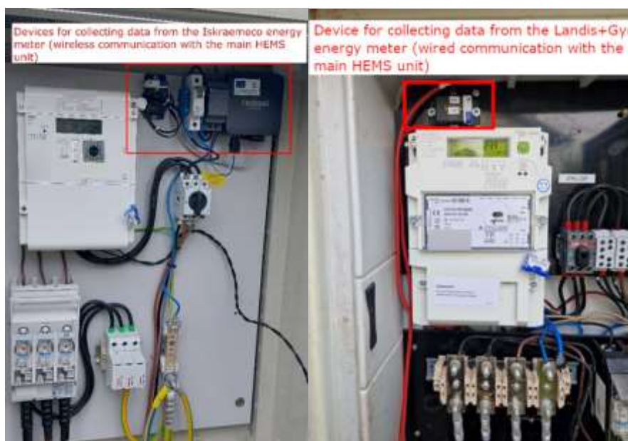
Figure 2: Iskraemeco and Landis+Gyr connection to P1/I1 user interface
